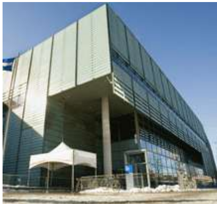
The Bibliothèque et Archives nationales du Québec on Montreal's Berri Street has been shedding its frosted glass panels almost since it opened in 2005. (Paul Chiasson/Canadian Press)
