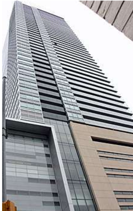
A missing pane of glass can be seen about halfway up the Festival Tower at King and John streets in Toronto. The piece of glass fell from a 27th-floor balcony on Tuesday night. Andrew Lupton/CBC
